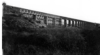
High Bridge over the Appomattox River near Farmville, Virginia. Photographed in 1865 by Timothy H. O'Sullivan during repairs following its burning during the war.
